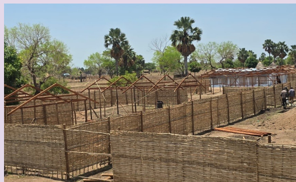
Photo: Ongoing construction of CTU structures at Pharqueng PHCC using local timber and woven fencing panels.
